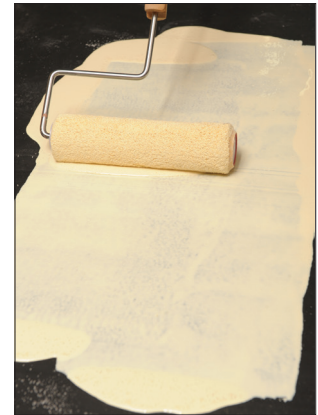
Apply EPDM Primer with brush, roller or spray. Allow to dry before applying the Sealoflex System
